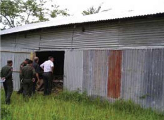
Another example is the “storage building” in one of the Brigades. The “building” is made of a wooden structure with corrugated iron sheets used both as walls and as the roof. There is absolutely no ventilation.
